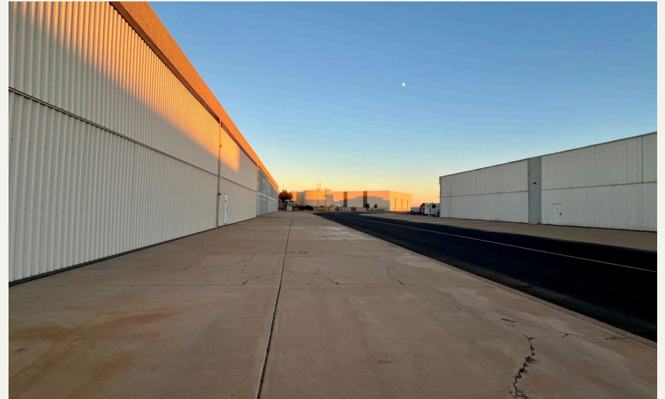
Hangar exterior and paved approach
